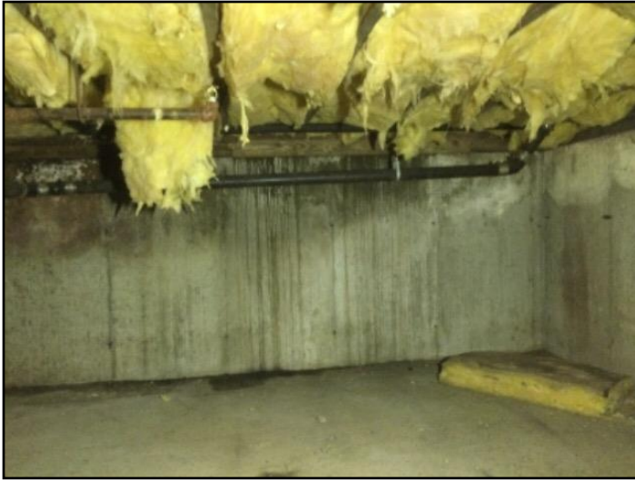
Fallen insulation in the floor structure
