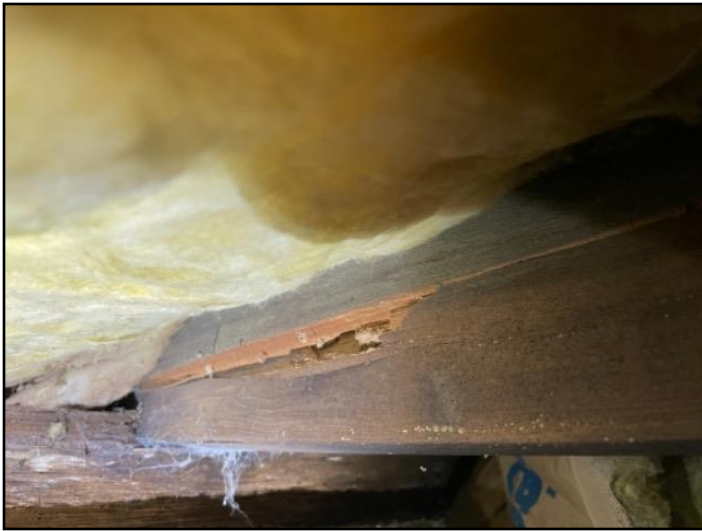
Evidence of insect damage noted
