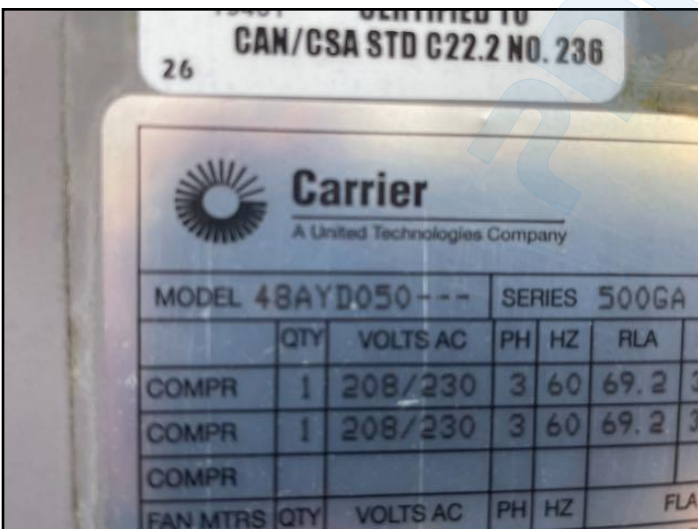
Packaged heating and cooling unit
