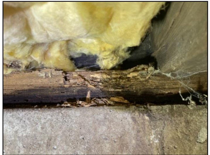
Evidence of insect damage noted
