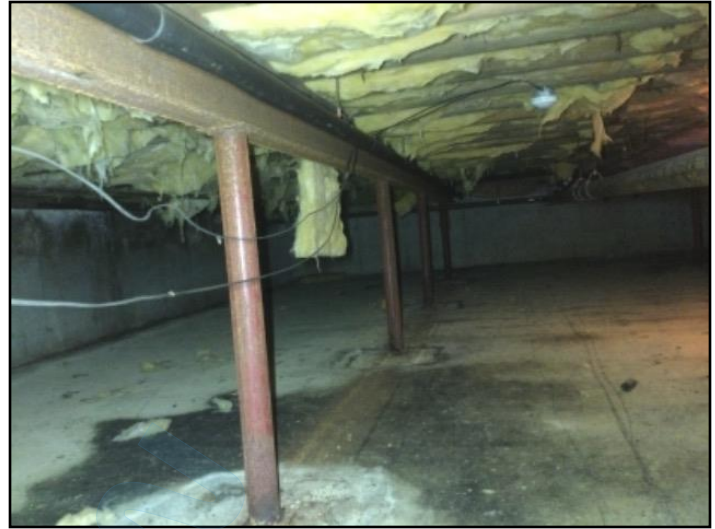
Fallen insulation in the floor structure
